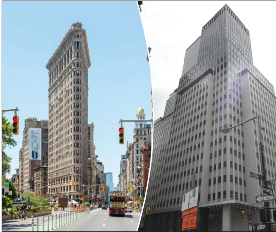
Office to resi conversions are still rare but buildings like the Flatiron and 222 Broadway are making the leap. Helayne Seidman, Getty
